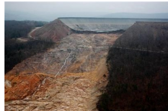
Taum Sauk Reservoir Failure
