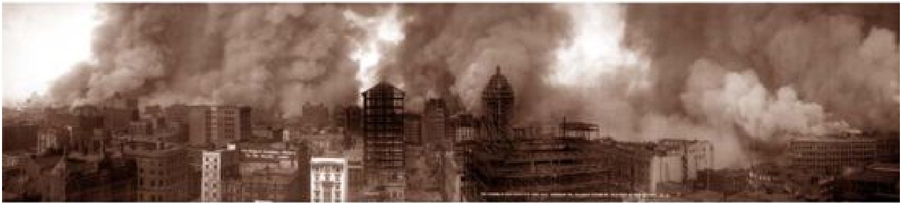
1906 San Francisco Earthquake
