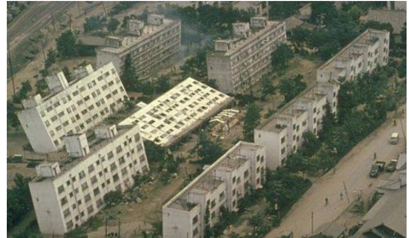
Liquefaction results after earthquake in Japan
