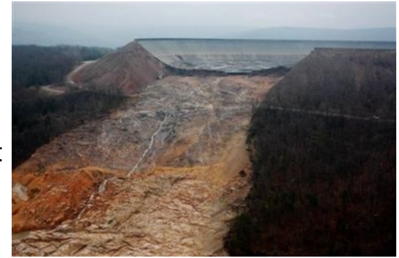
Taum Sauk Reservoir Failure
