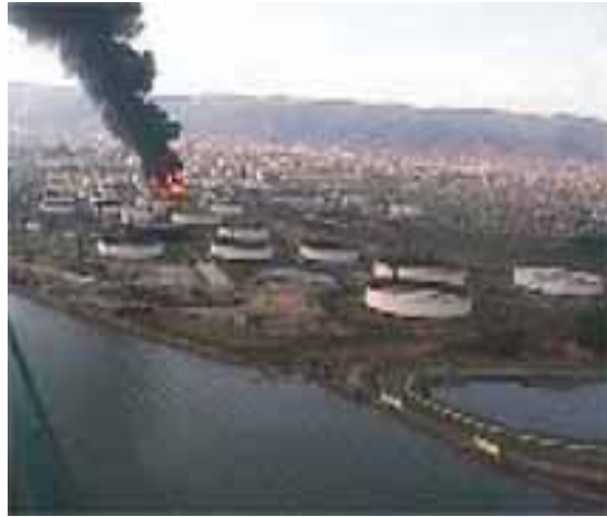
1999 Izmit, Turkey, earthquake
